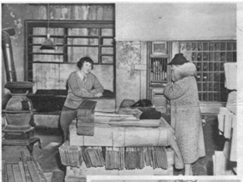
Shaping up – Ralstonites check up on progress of reconstruction of the building's interior. The structure was built in 1776 as a general store. Fourth-class post office was established in 1892. Sunday Evening News January 11, 1942.
